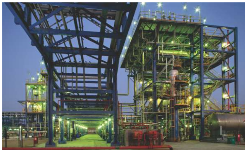
Raageshwari Gas Terminal, Barmer, Rajasthan
