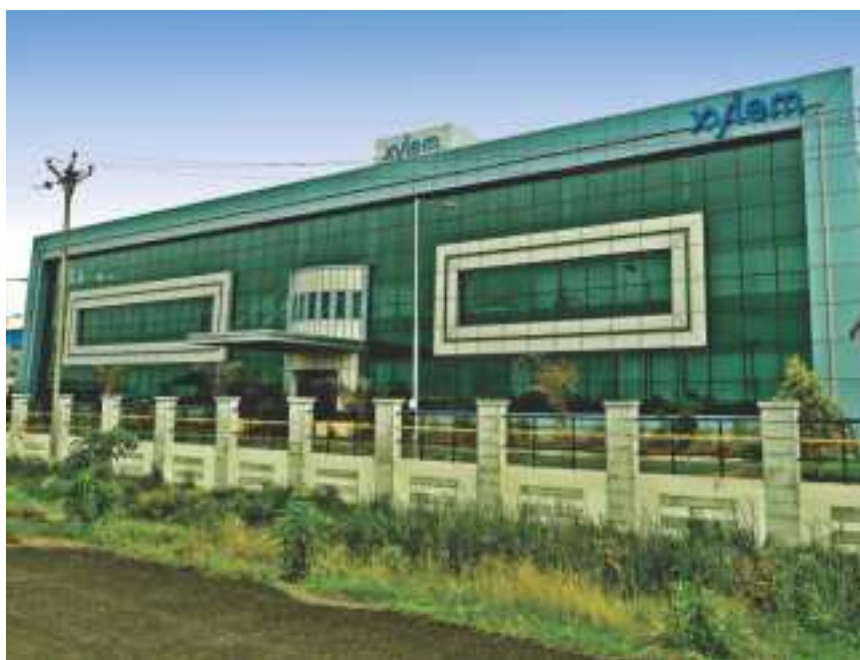
Manufacturing & Pump Testing Facility, Vadodara
