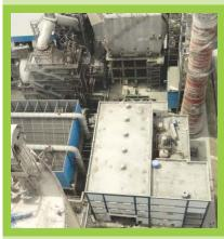
Study of 10 electrostatic precipitators through process simulation and incorporation of improvements to meet the revised emission norms of 30mg/Nm<sup>3</sup>
