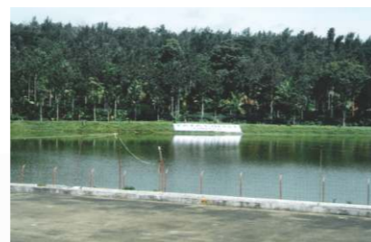
Rainwater harvested in tanks
