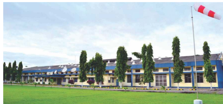
The dust extraction system has come as a breath of fresh air at Kellyden
