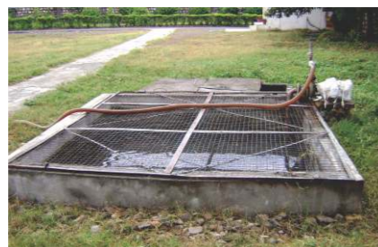
Underground tanks for collecting wastewater
