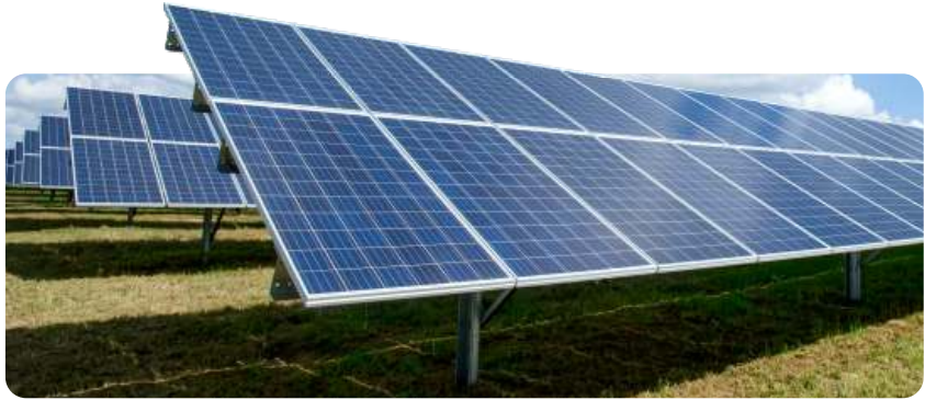
Solar panels installed at Ambattur, Chennai facility
