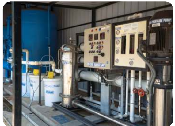
Water treatment plant at Ambattur, Chennai facility
