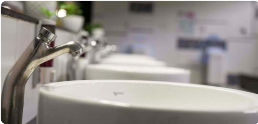
Sensor based taps installed in the restrooms of all major facilities.
