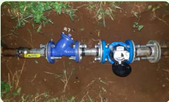
IoT water meters installed at Dighi campus, Pune
