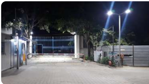
LED powered peripheral lighting at KIADB, Bengaluru facility
