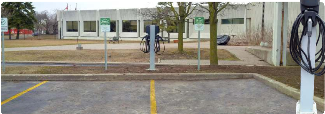
EV charging stations at Toronto, Canada
