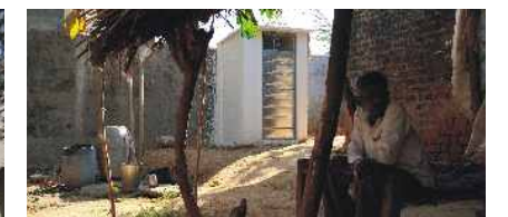
Sanitation facilities built for surrounding village homes ensure a hygienic environment
