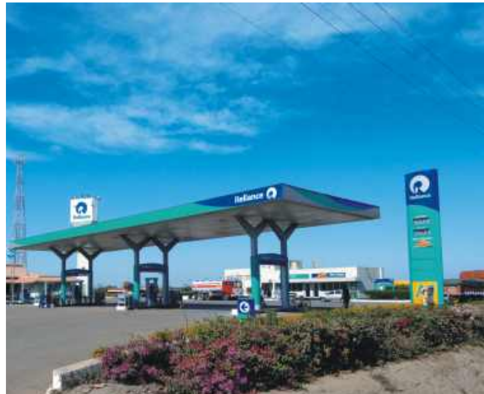
RIL's Petrol Outlets designed with real-time automation, delivering enhanced customer experience.
