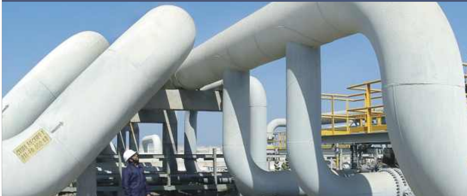
Jamnagar Marine Tank Farm Crude Receiving Center
