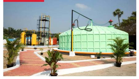
About 8 tons of food waste is converted to 1000 m<sup>3</sup> of bio-gas and 4 tons of fertiliser. The bio-gas is converted into 400 m<sup>3</sup> of compressed natural gas to run buses, tractors and generators.
