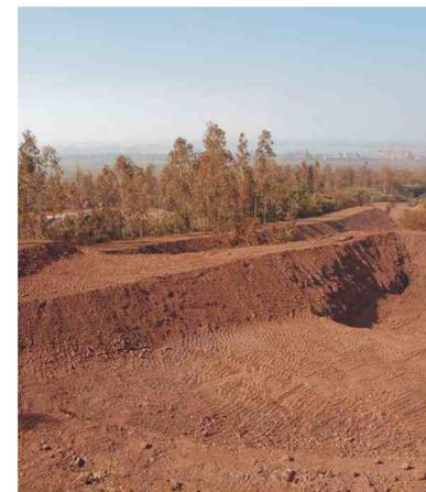
off to check dams so that silt deposits are collected and removed during summers. Collected sediments are segregated and useful products are recycled and used for strengthening bunds to level the low-lying areas. During rainy season water from check bunds is collected both from upstream and downstream and analysed for physical and chemical parameters.
