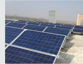
Rooftop solar plant at Evolve - the GnNxt IT park in MWC, Jaipur
