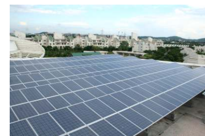
Rooftop solar PV at 'Evolve'
