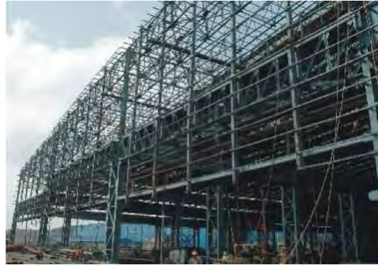
Efficient logistics & effective site management minimises material wastage
