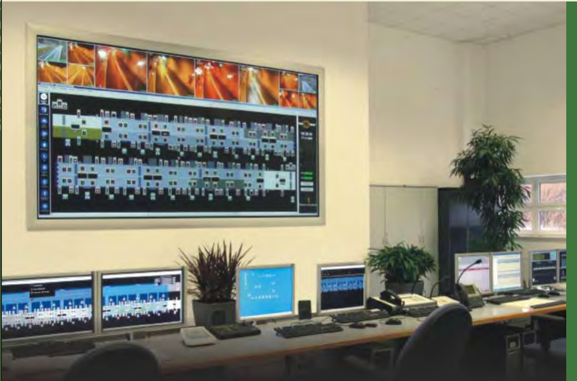
The Supervisory Control And Data Acquisition (SCADA) system supplied by L&T for offshore operations to ONGC
