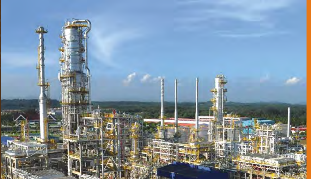
Stacks at Melaka Refinery, Malaysia
