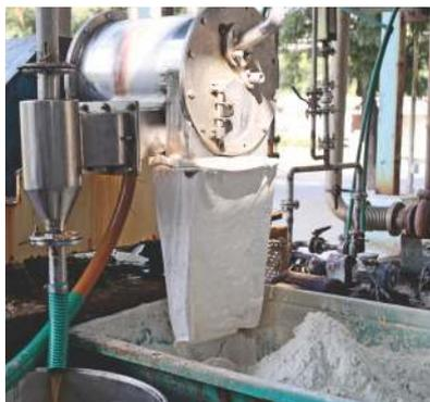
Our Santej unit is a Zero Liquid Discharge (ZLD) unit. In 1998, the unit invested in ZLD technology to set up an Effluent Treatment Plant (ETP) with a capacity to treat 17,500 cubic meter of textile effluent per day. In FY 2014, we installed Mechanical Vapour Recompression Evaporation (MVRE) plants in the effluent recycling system for low cost evaporation and recovery of salts dissolved in the effluents.
